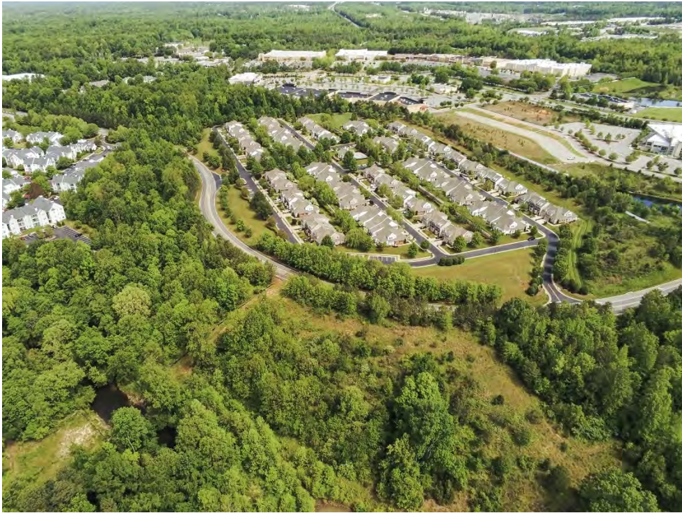
Bailey Bridge Connector at Brad McNeer Parkway Before Photo
