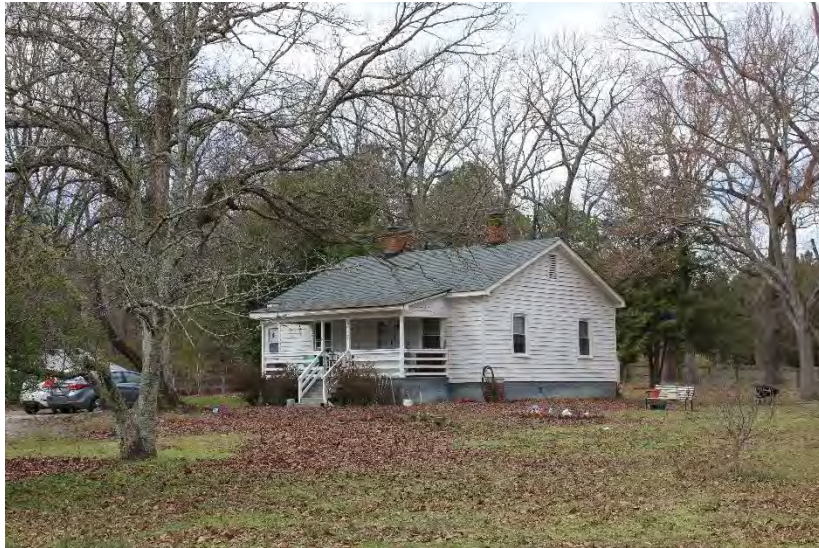
View of house looking west-northwest
