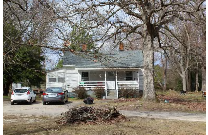
View of house looking north-northwest
