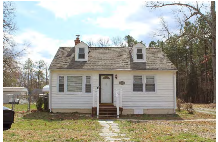
View of house looking south-southeast
