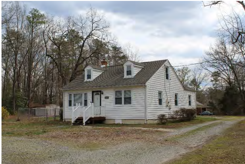
View of house looking southeast
