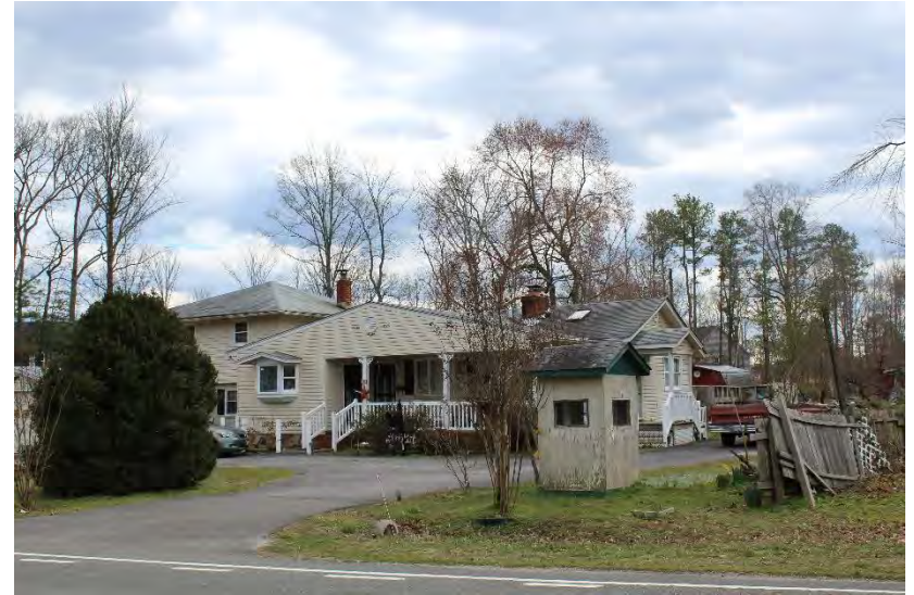
View of house looking southeast
