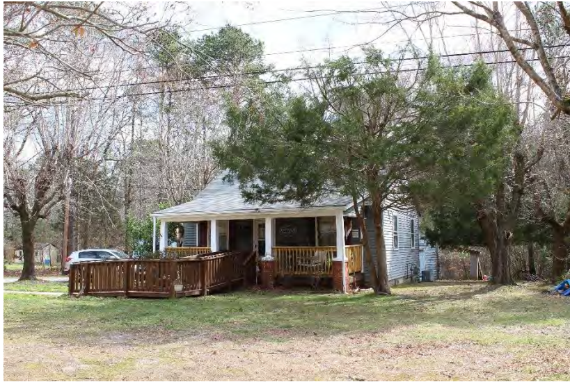
View of house looking southeast
