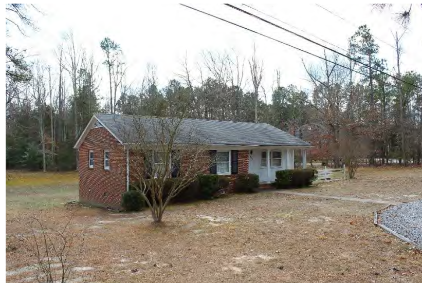
View of house looking southwest
