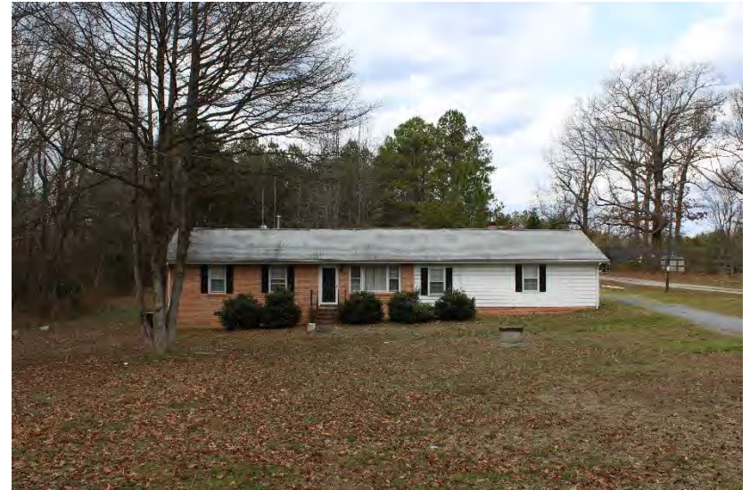
View of house looking north-northwest
