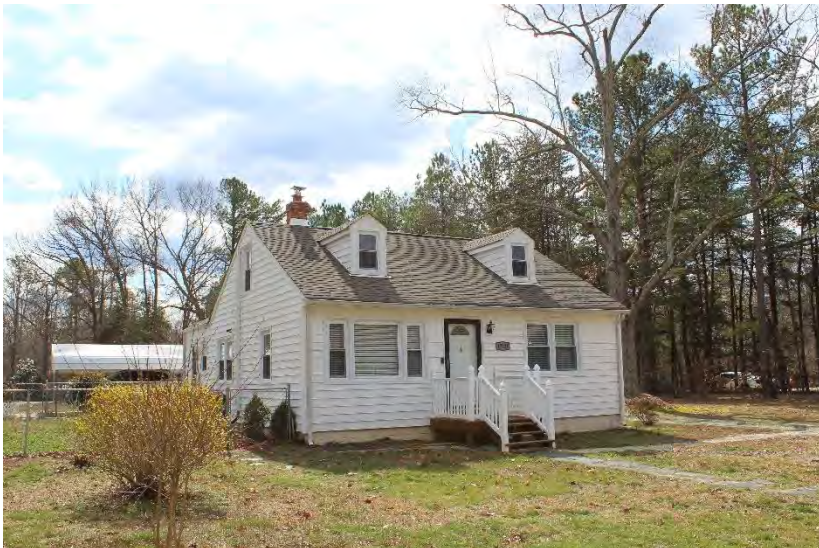
View of house looking south-southwest
