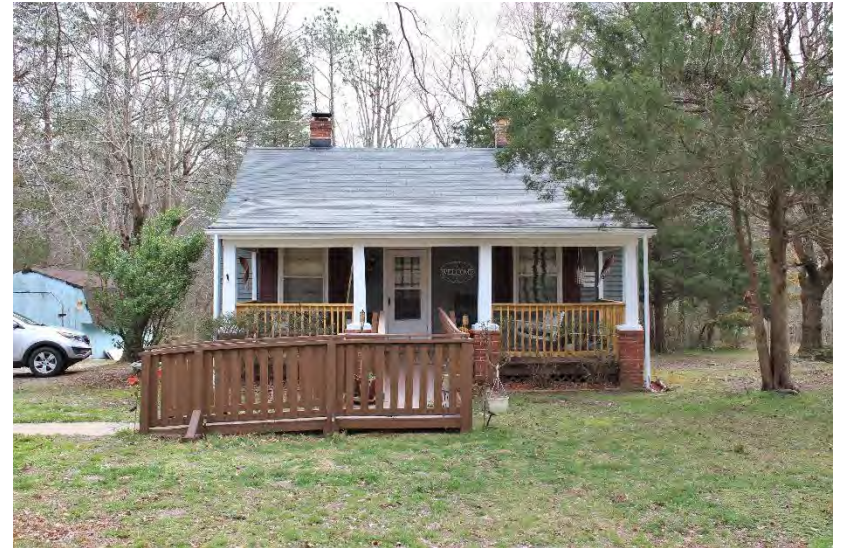
View of house looking south-southeast
