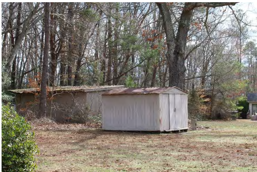
View of outbuildings looking southeast
