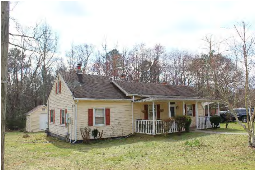
View of house looking southwest
