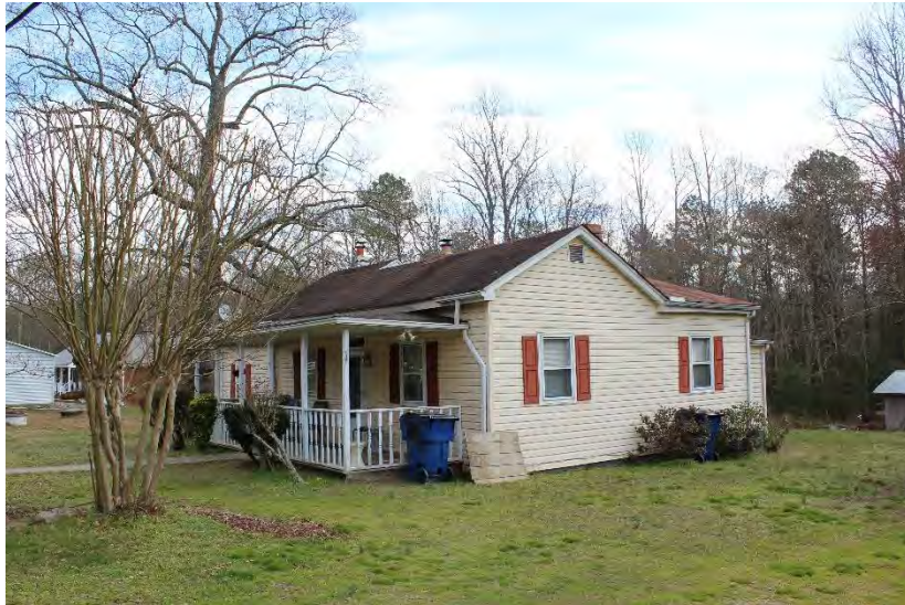
View of house looking southeast
