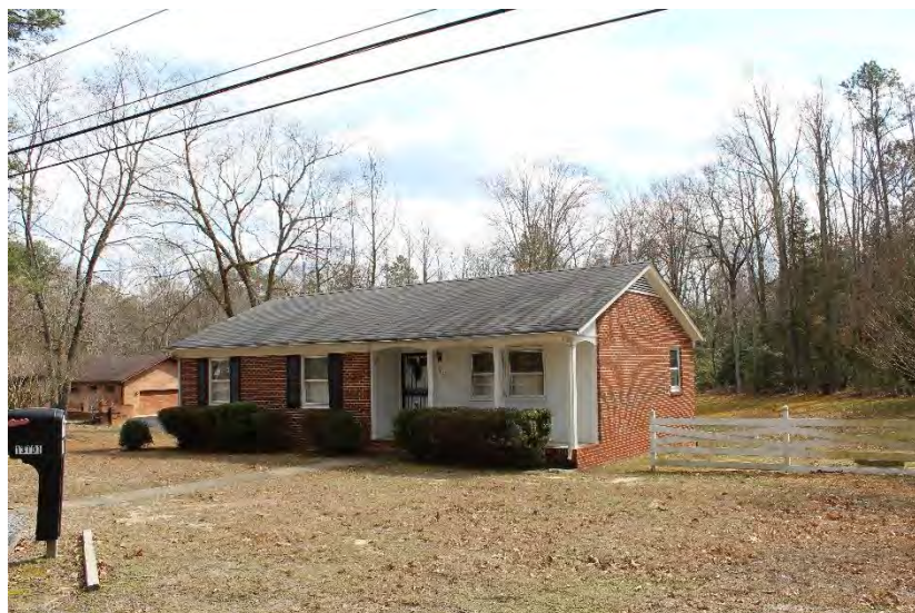
View of house looking southeast
