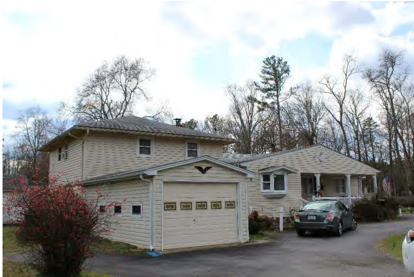
View of house looking southwest
