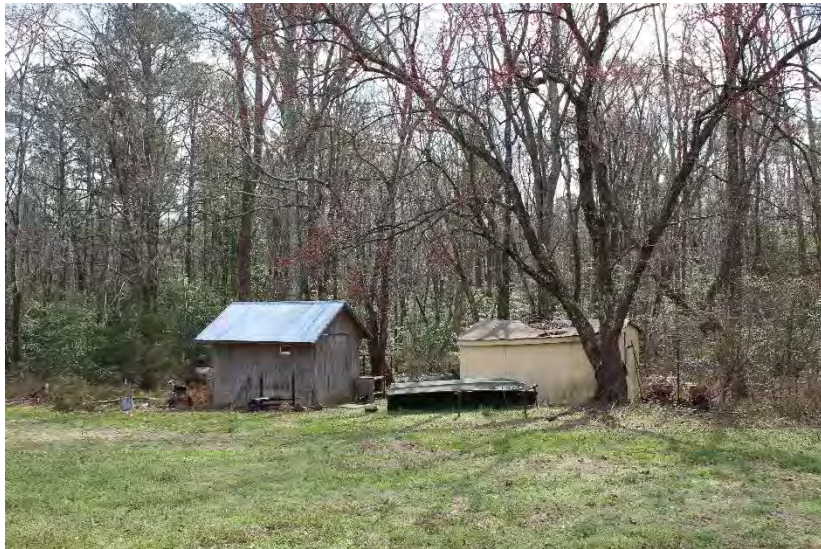
View of outbuildings looking southeast
